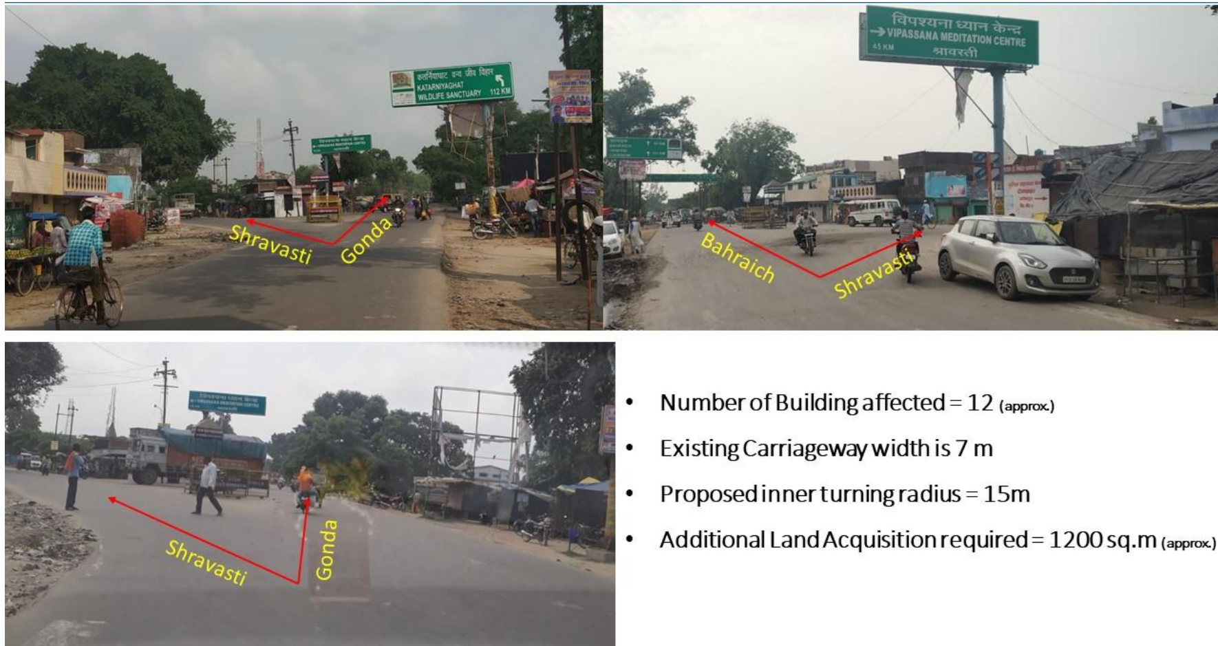
Figure 3.2: Existing connectivity between SH-30 and NH-730 at Y junction at Chainage 0.000Km
