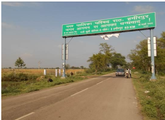
Start of Project Road at Km 74+550 SH-42
