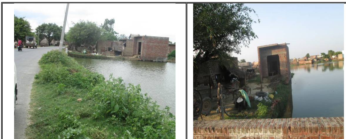
Existing status of the pond at Km 61+500 (RHS) at Wahpurpatti
